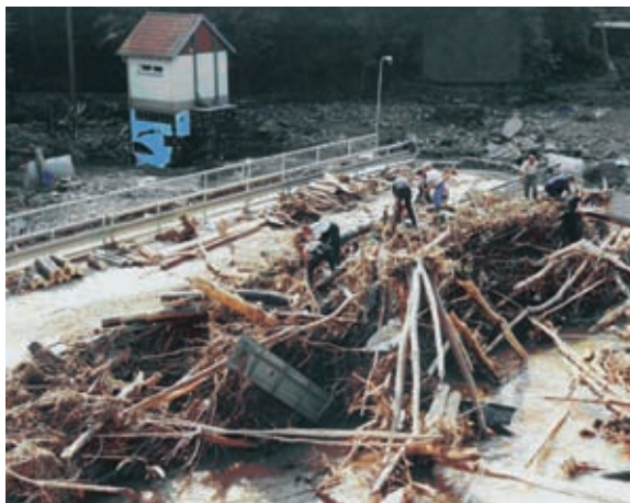
Fig. 4: Complete erosion of the railroad embankment in the valley of the river Müglitz. The exposed old retaining wall, which used to give the stream a much wider bed, is noteworthy (photo: LTV [State Dam Management Office], 2002).
