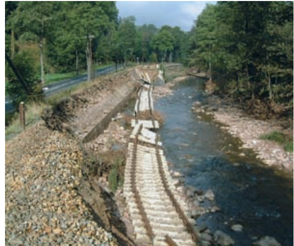
Fig. 4: Complete erosion of the railroad embankment in the valley of the river Müglitz. The exposed old retaining wall, which used to give the stream a much wider bed, is noteworthy (photo: LTV [State Dam Management Office], 2002).
