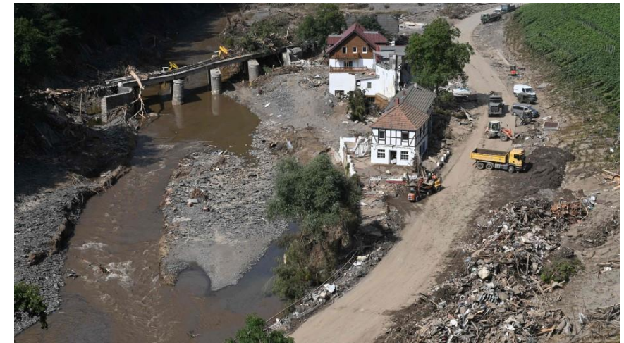
Massive flooding on 14 July 2021 in the Ahr valley caused fatalities and massive damage (faz.net)
